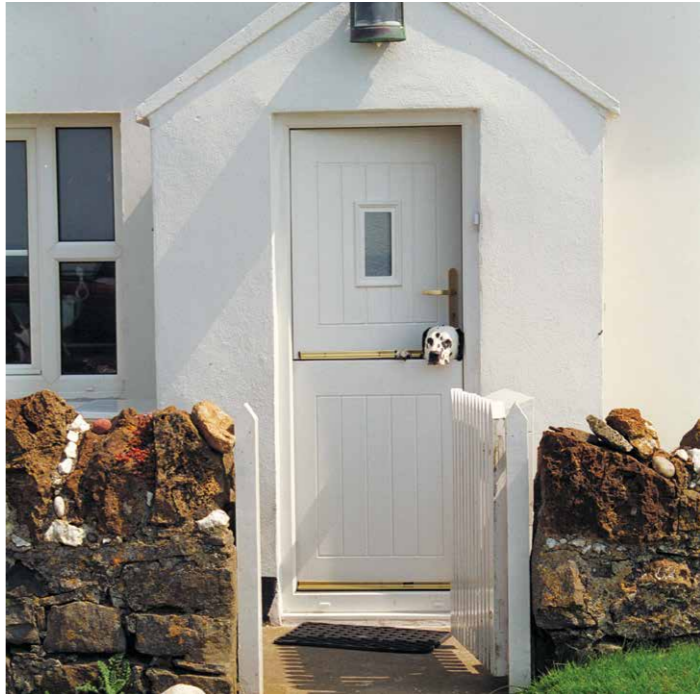
20 YEAR HISTORY. The Stable Door pictured here was installed on a coastal property on the Isle of Man 20 years ago and still looks good today.
